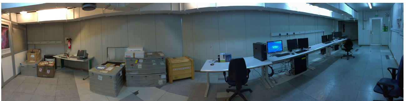
Figure 3. The AstraLux Sur boxes and control computers inside the NTT local control room.
